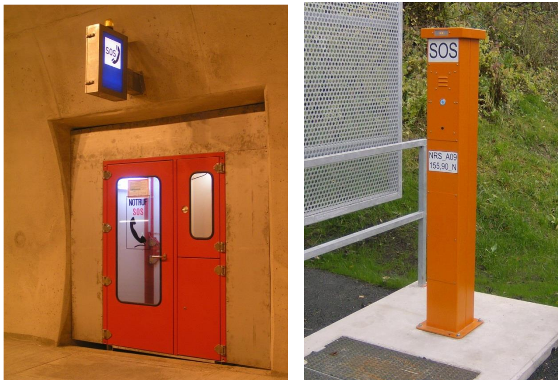
Fig. 2 Emergency call unit located inside the tunnel and at lay-bys and emergency call column located at tunnel portals
